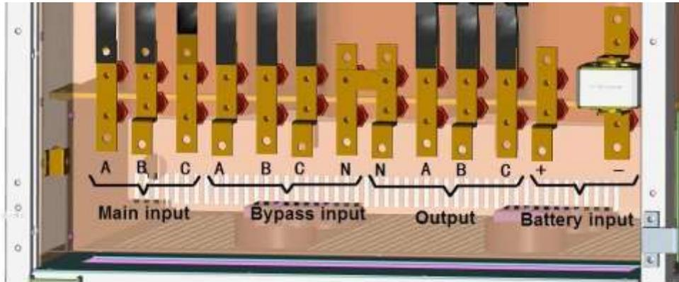
Figure 3-10: Wiring Terminals of 80 ~120KVA UPS
