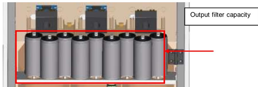
Figure 2-17: 60KVA UPS AC Output Capacity Module
